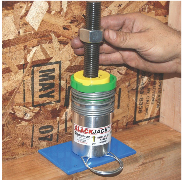
2. Place color coded washer and spin nut down hand tight.
